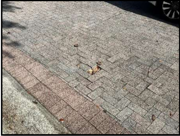
Figure 3 – Missing paver by sport courts parking area
