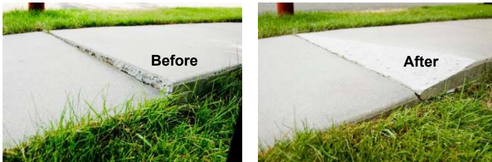
Figure 10: Precision Sidewalk Safety Work Example
