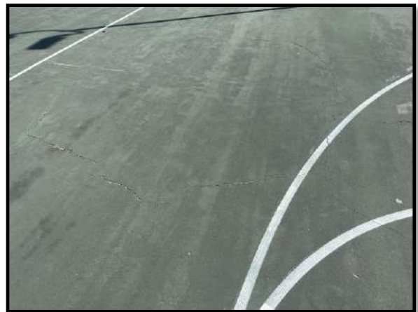
Figure 2 – Cracks at basketball court
