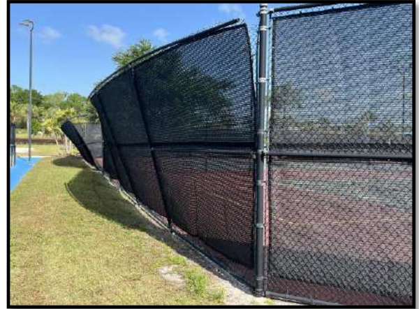
Figure 2 – Falling fence at pickleball/tennis courts
