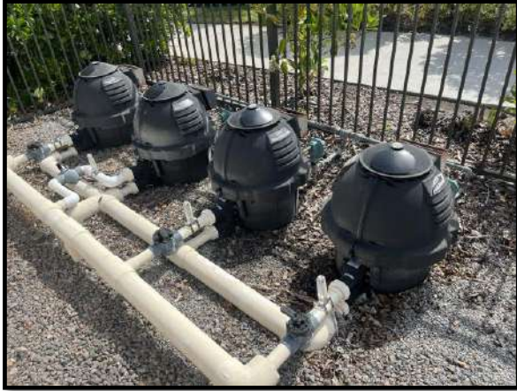
Figure 1 – Pool heaters
