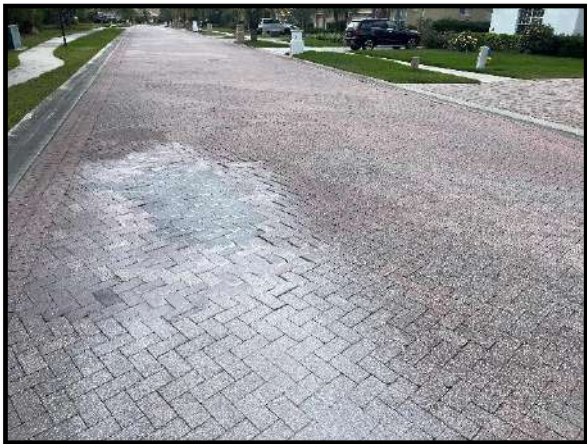
Figure 11 – Paver settlement at Cory Lake Drive
