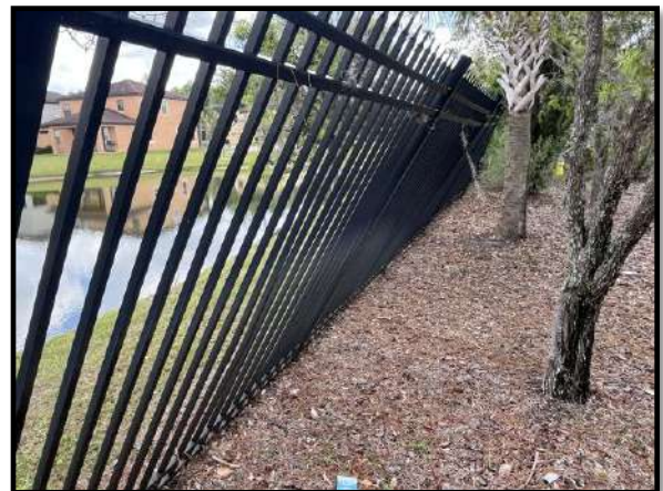
Figure 2 – Leaning section of aluminum fence
