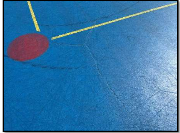
Figure 4 – Court deterioration
