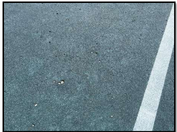
Figure 8 – Holes in tennis court surface
