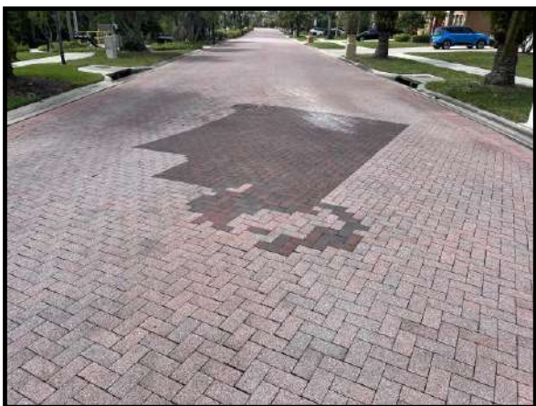
Figure 7 – Replaced pavers at Cory Lake Drive
