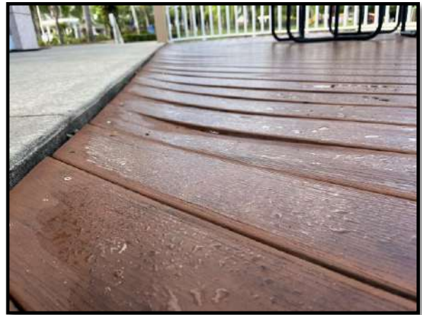
Figure 2 – Warped deck board
