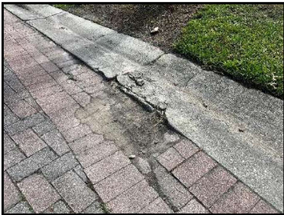
Figure 1 – Concrete curb damage at Cory Lake Drive
