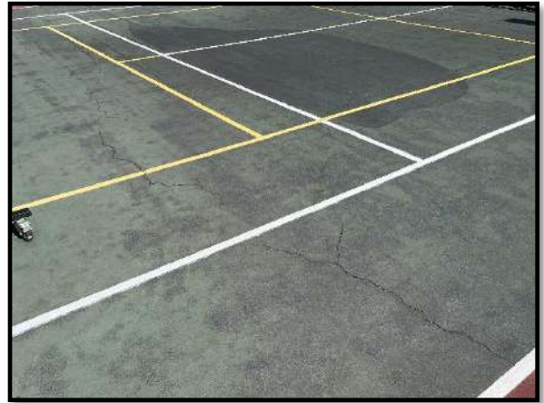
Figure 6 – Large pickleball/tennis court cracks
