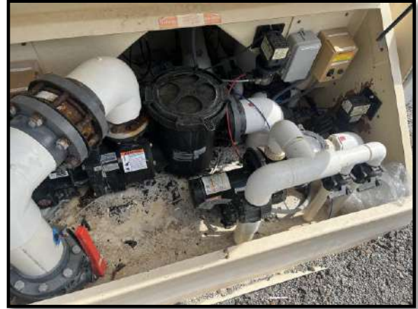
Figure 2 – Pool pumps and chlorinators
