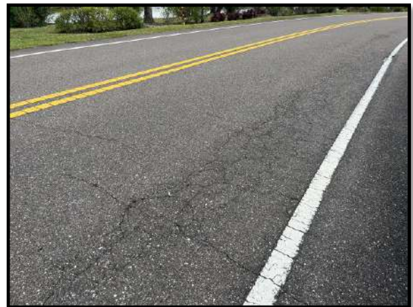
Figure 2 – Alligator cracking at Cory Lake Drive
