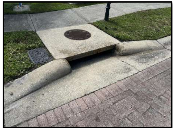
Figure 2 – Typical street stormwater inlet
