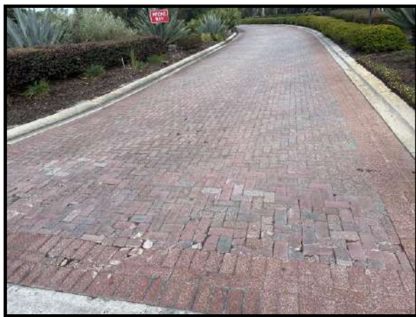
Figure 1 – Damaged pavers at southeast entrance
