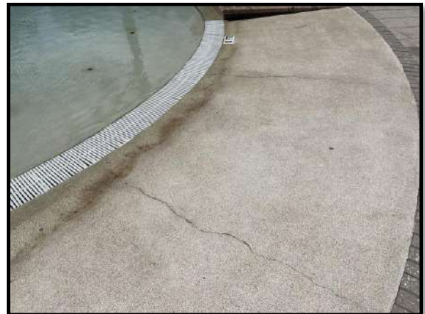
Figure 2 – Plaster finish cracks
