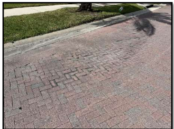
Figure 8 – Paver settlement at Martinique Isle Drive
