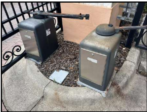
Figure 1 – Typical swing gate operators
