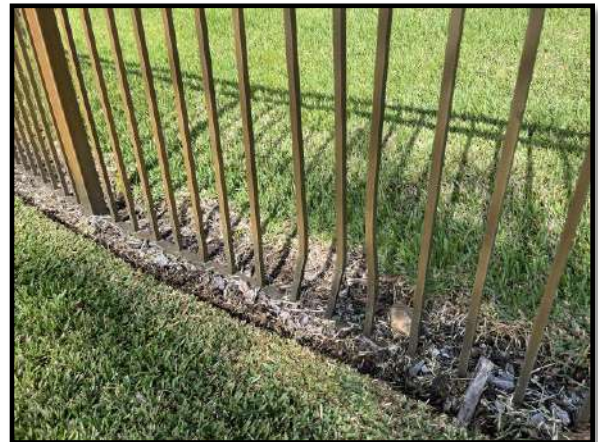
Figure 2 – Isolated fence damage by water slide
