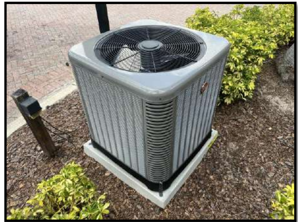
Figure 2 – New condensing unit at gatehouse
