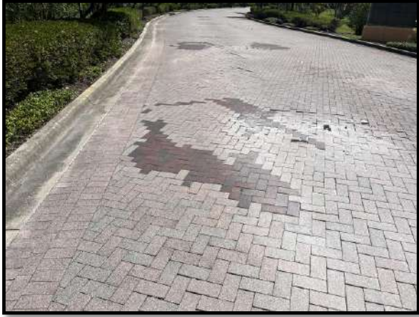
Figure 9 – Damaged pavers at Cory Lake Boulevard
