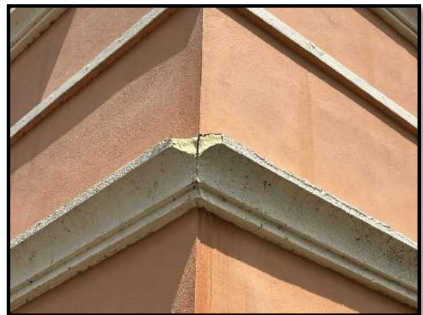
Figure 2 – Isolated entrance monument damage
