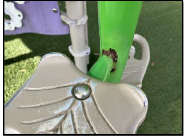
Figure 2 – Playground rust and finish deterioration
