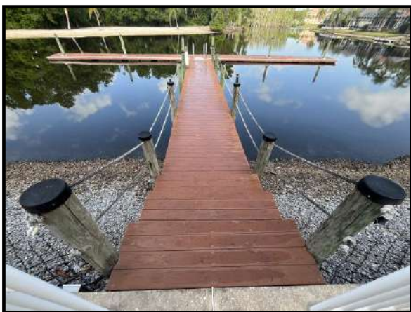
Figure 1 – Overview of docks
