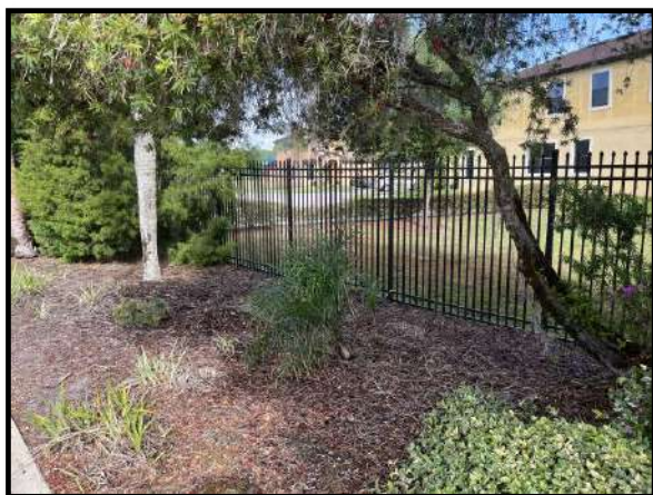
Figure 1 – Aluminum fence at southeast entrance
