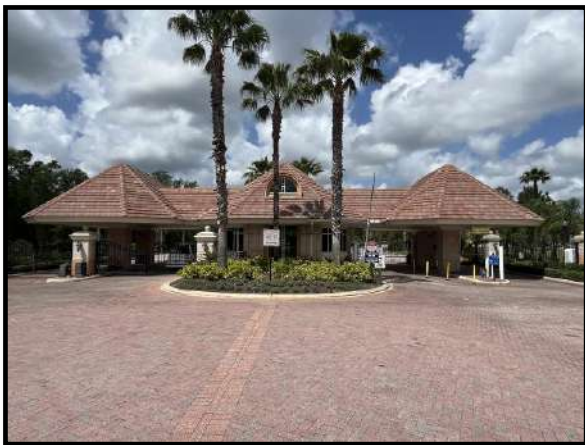
Figure 5 – Southeast gatehouse roof overview
