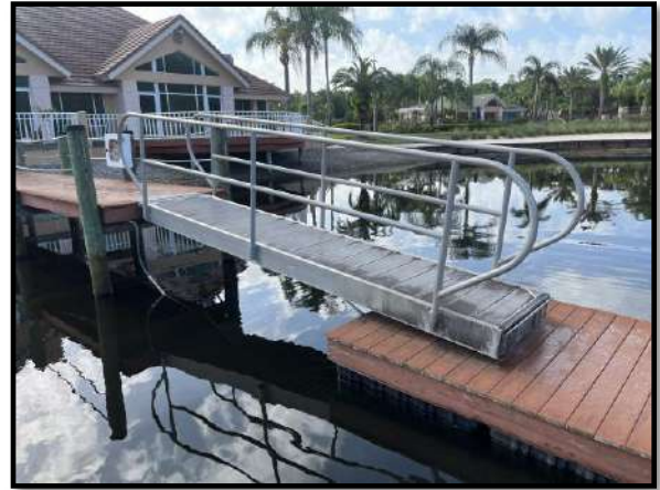
Figure 4 – Gangway between docks
