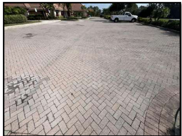
Figure 2 – Pavers at Beach House parking area
