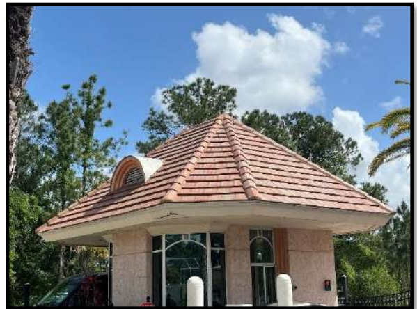
Figure 4 – Tile roof at northwest gatehouse
