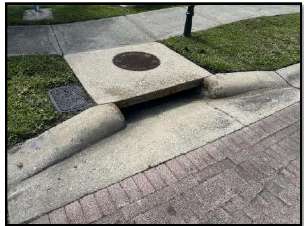
Figure 2 – Typical street stormwater inlet
