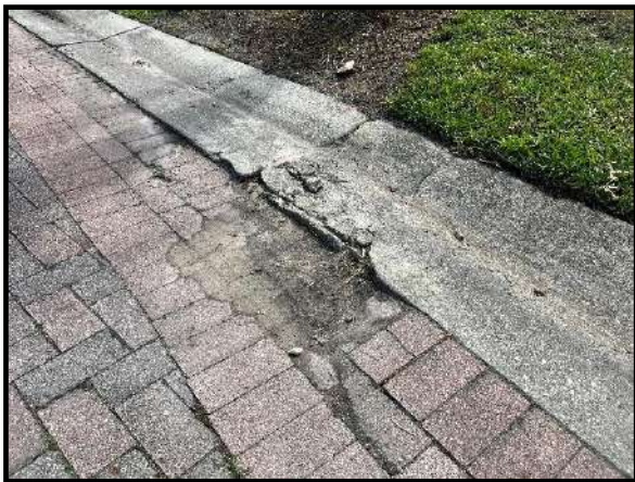
Figure 1 – Concrete curb damage at Cory Lake Drive
