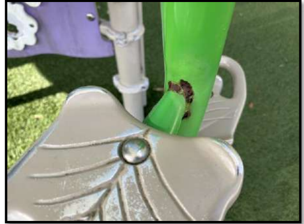
Figure 2 – Playground rust and finish deterioration
