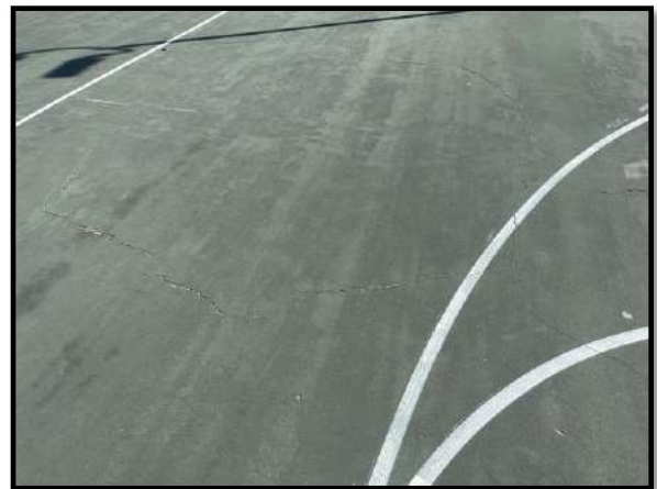
Figure 2 – Cracks at basketball court
