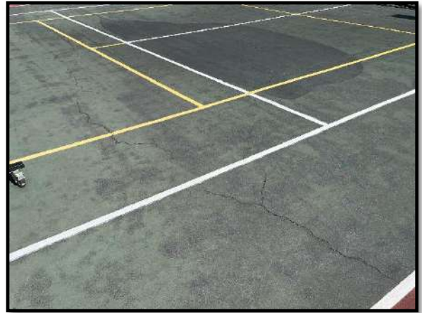
Figure 6 – Large pickleball/tennis court cracks
