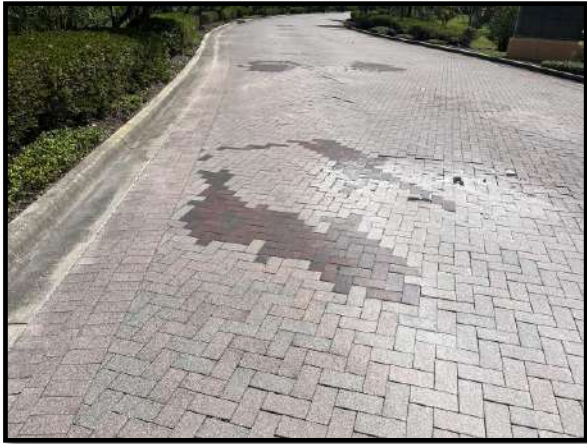
Figure 9 – Damaged pavers at Cory Lake Boulevard
