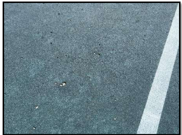
Figure 8 – Holes in tennis court surface
