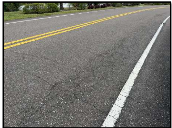
Figure 2 – Alligator cracking at Cory Lake Drive
