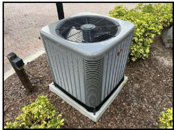
Figure 2 – New condensing unit at gatehouse
