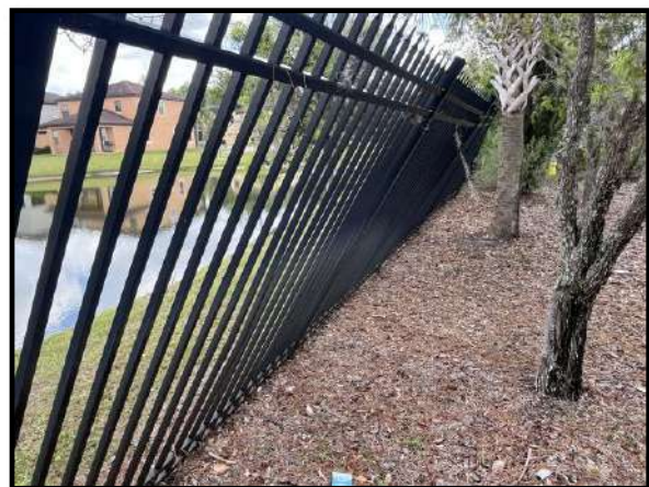
Figure 2 – Leaning section of aluminum fence
