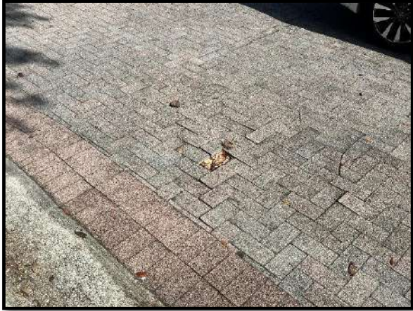
Figure 3 – Missing paver by sport courts parking area
