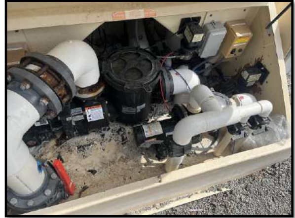
Figure 2 – Pool pumps and chlorinators
