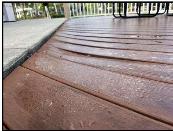
Figure 2 – Warped deck board
