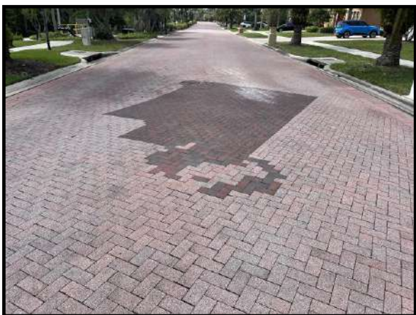
Figure 7 – Replaced pavers at Cory Lake Drive
