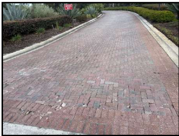
Figure 1 – Damaged pavers at southeast entrance
