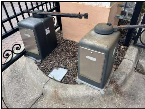
Figure 1 – Typical swing gate operators
