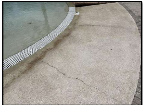
Figure 2 – Plaster finish cracks
