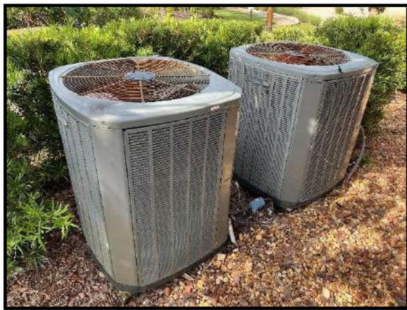
Figure 1 – Condensing units at the Beach House
