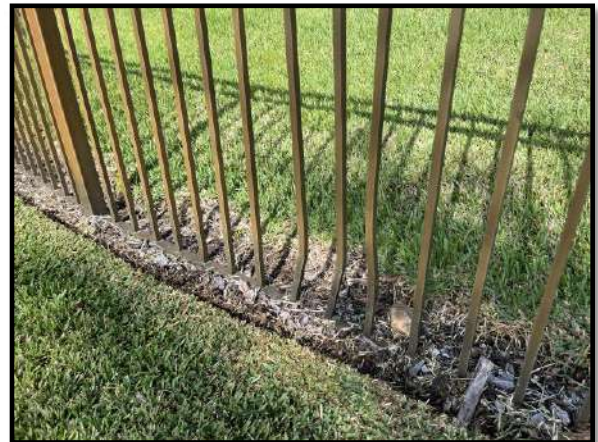
Figure 2 – Isolated fence damage by water slide
