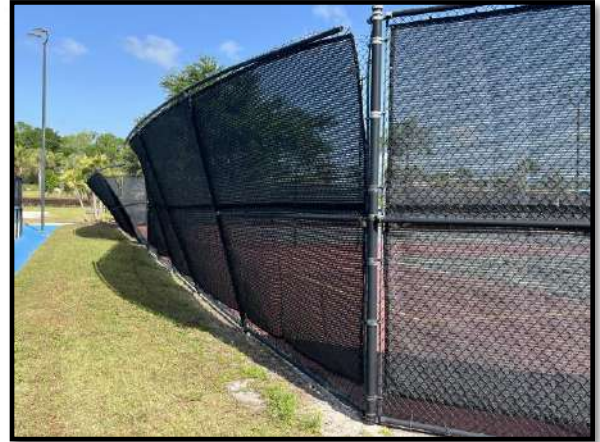
Figure 2 – Falling fence at pickleball/tennis courts
