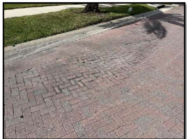
Figure 8 – Paver settlement at Martinique Isle Drive
