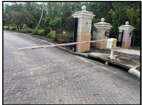
Figure 2 – Typical lift gate operators
