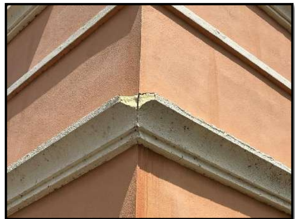
Figure 2 – Isolated entrance monument damage
