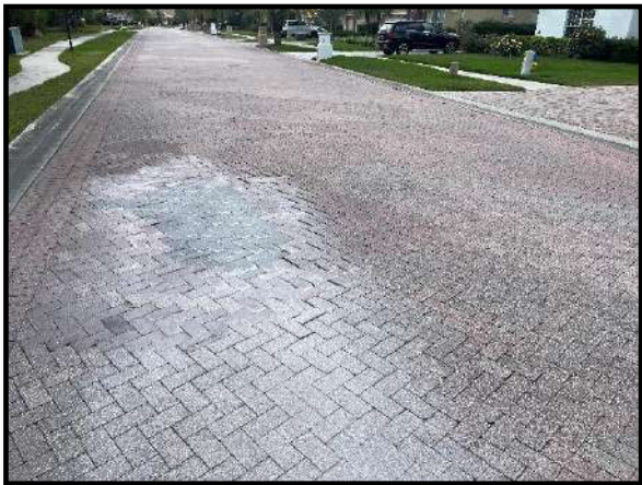
Figure 11 – Paver settlement at Cory Lake Drive
