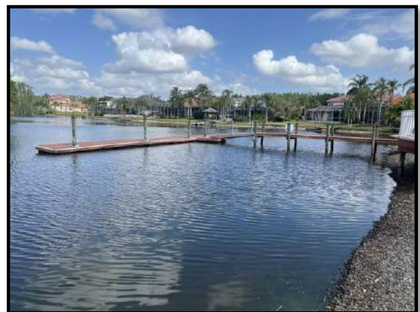
Figure 2 – Docks and pilings with gangway
