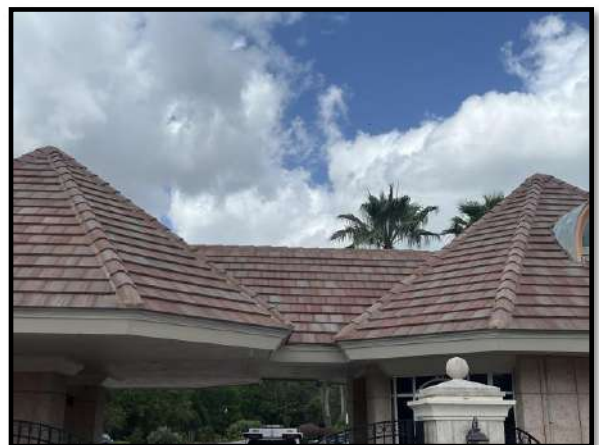
Figure 6 – Roof tiles at southeast gatehouse
