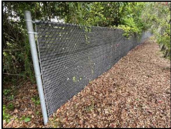
Figure 1 – Chain link fence overview
