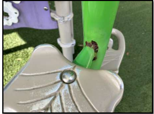
Figure 2 – Playground rust and finish deterioration
