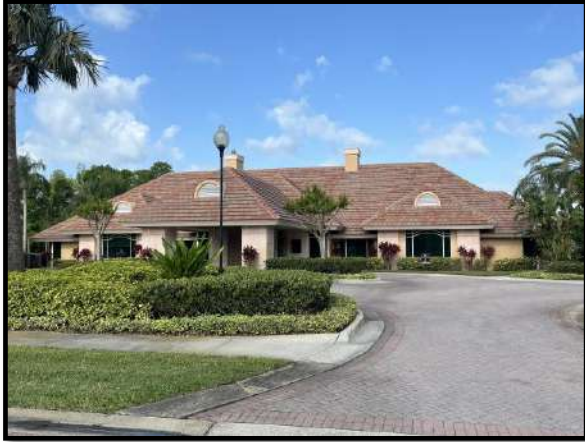
Figure 1 – Beach House roof overview
