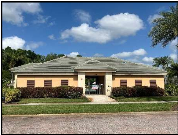
Figure 3 – Pool house tile roof
