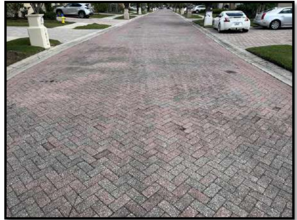
Figure 12 – Pavers overview at Cozumel Isle Drive
