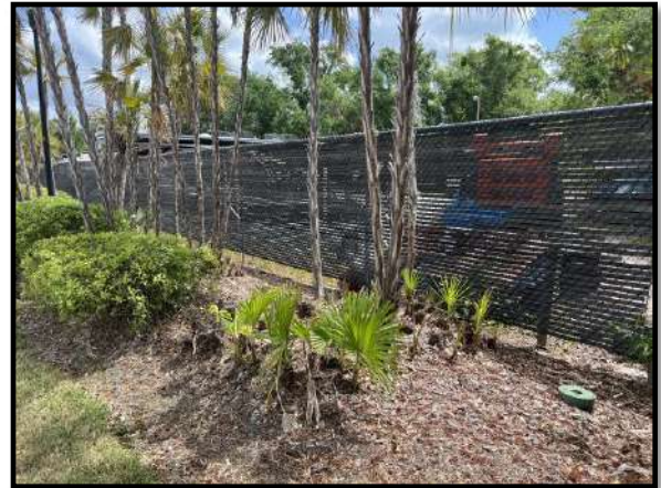
Figure 2 – Chain link fence
