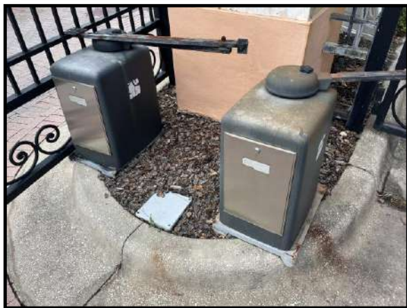
Figure 1 – Typical swing gate operators
