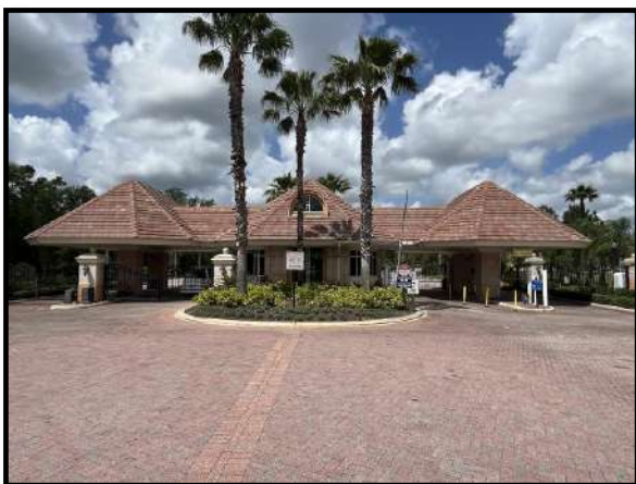
Figure 5 – Southeast gatehouse roof overview
