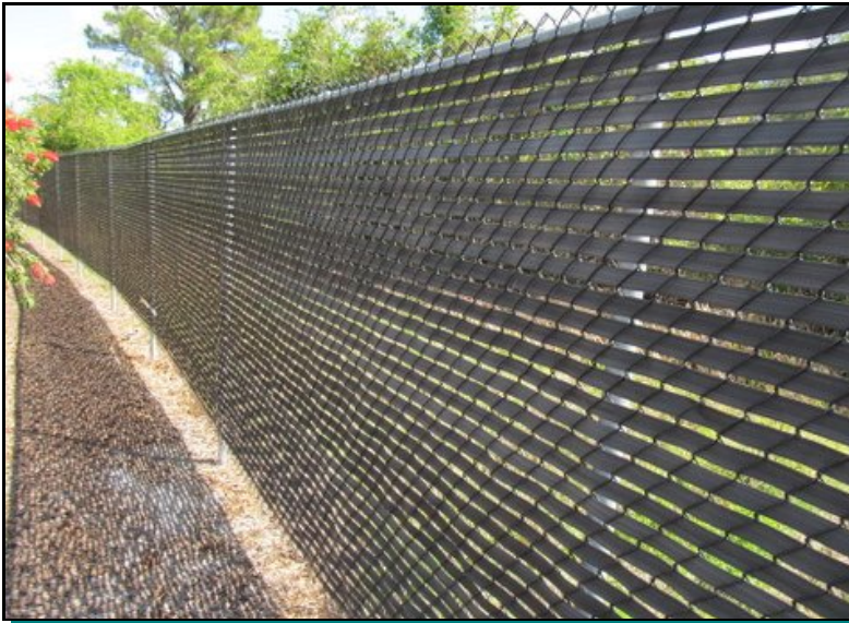
Chain link fence
