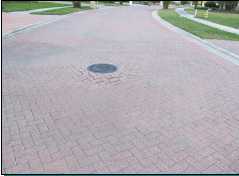
Paver settlement Maintain through the Operating Budget
