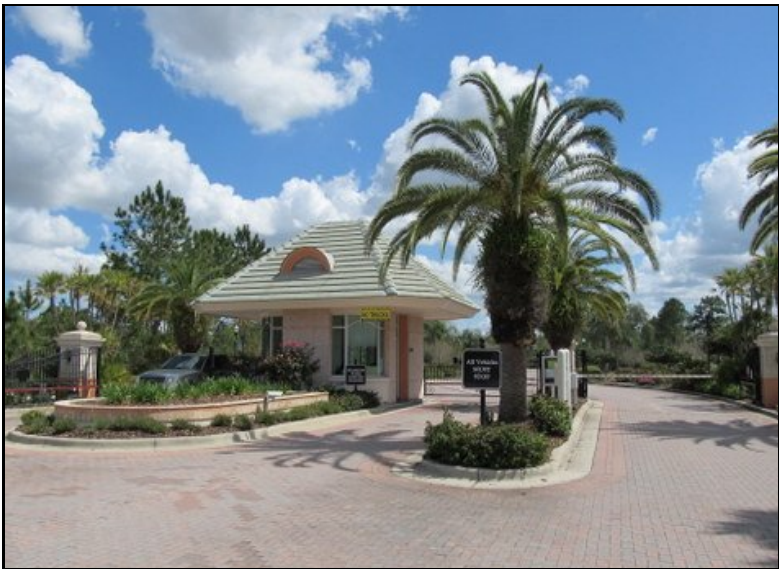
West gate house
