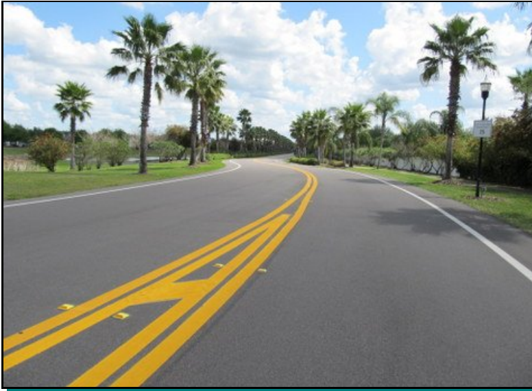
Cory Lake Drive asphalt pavement
