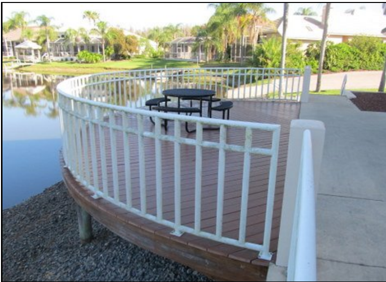
Beach house deck
