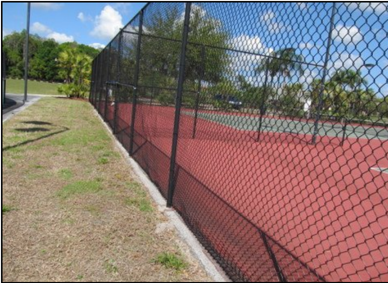
Tennis court fence
